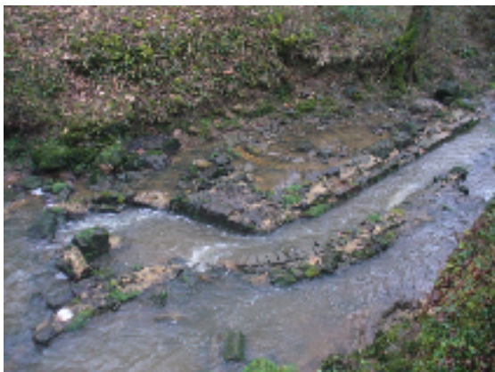
The site following winter 2012
