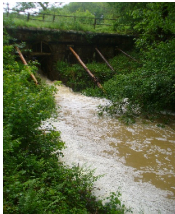
Overflow spillway in full flood
