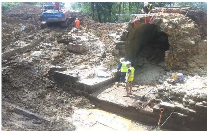
Southern Spillway and Barrel Arch July 2021
