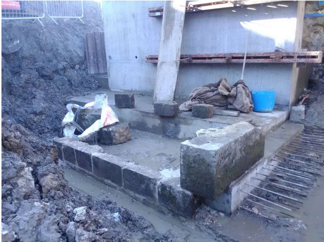
Red letter day of 8 th December, the first stones are rebuilt.
